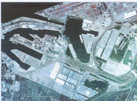
Overview RoRo-Terminal Bremerhaven
